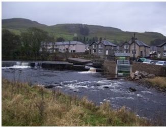
The wear at Settle with the screw and generator house
